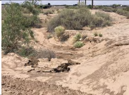
View of storm water discharge point on west side of site. Sediment has been removed from behind waddles.
