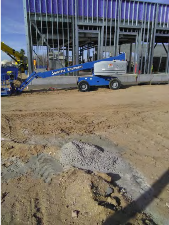
Site Walk Deficiency Photos - Concrete washout on ground SE corner of structure
