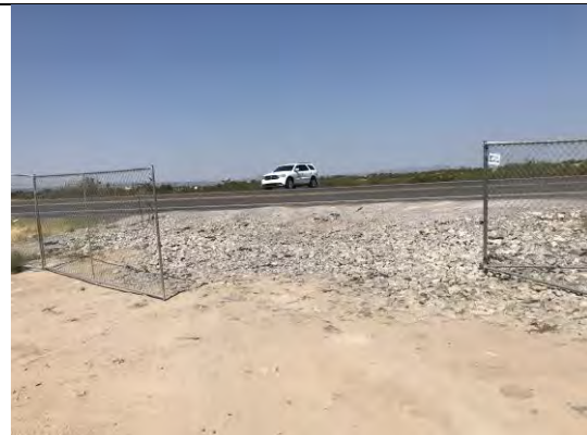
View of rock construction entrance.
