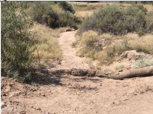
View of straw waddles across discharge point from site. Sediment behind waddles has been removed.
