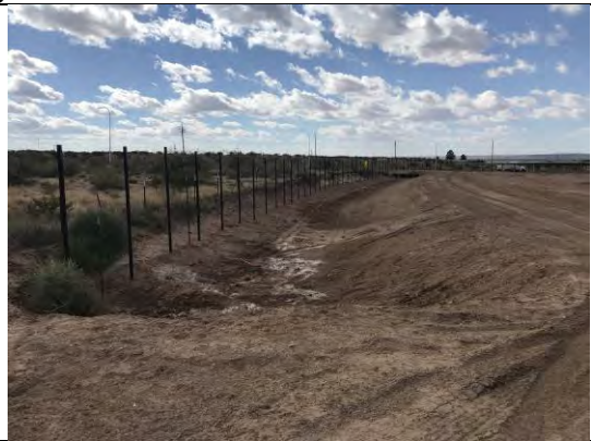
View of drainage swale 3. Swale has been regraded.
