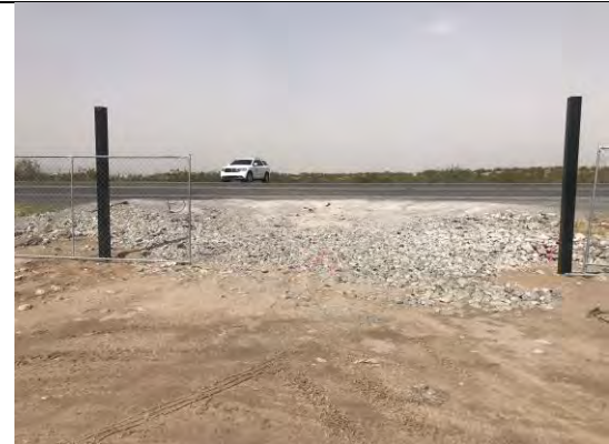
View of rock construction entrance.
