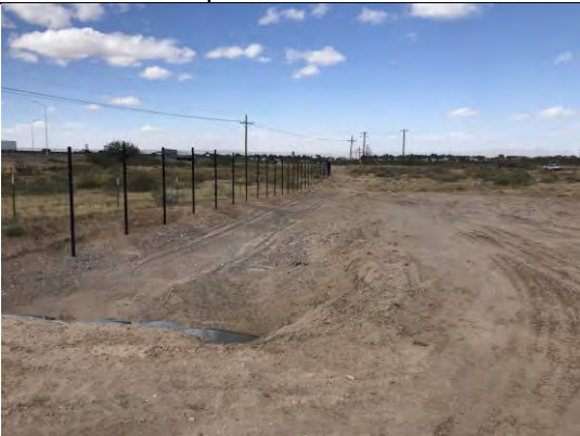
View of drainage swale No. 1.
