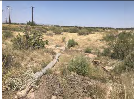
View of straw waddles on west side of site.
