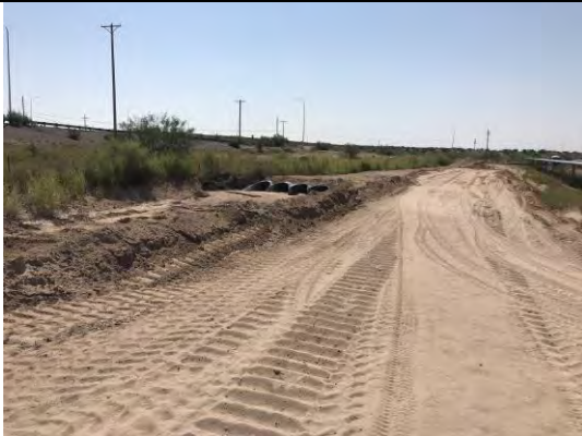
View of drainage swale No. 4. Berm has been built up on west edge of berm.
