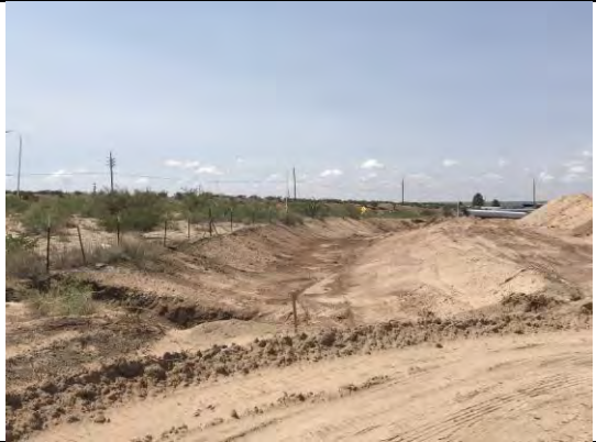
View of drainage swale No. 3 on southeast corner of site.
