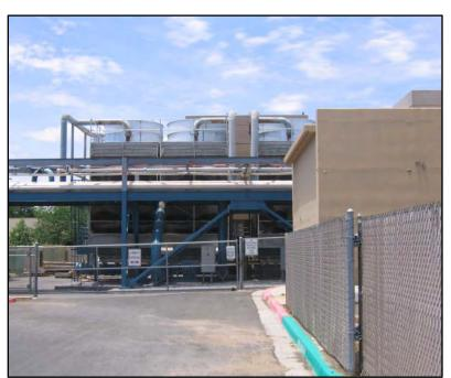
Figure 11. Cooling Towers behind Central Plant (NG-Fired Turbines are within Building on the Right Side).
