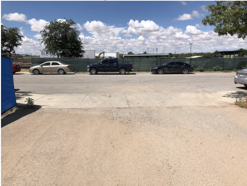
Site Walk Deficiency Photos - West entrance Trackout
