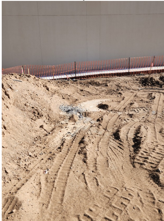
Site Walk Deficiency Photos - CWO NE
