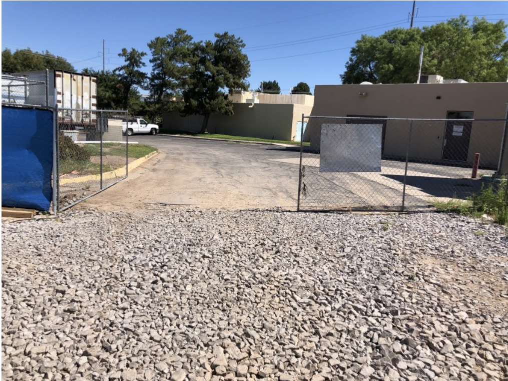
Site Walk Deficiency Photos - NE entrance
