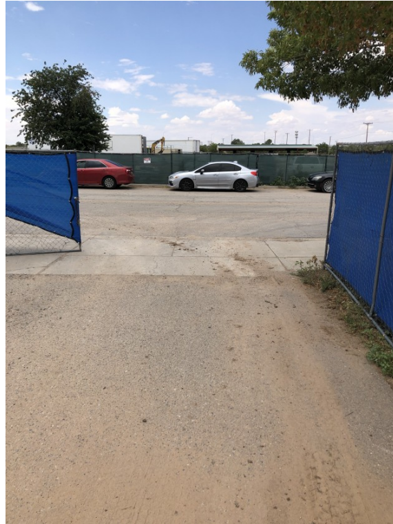
Site Walk Deficiency Photos - West entrance Trackout
