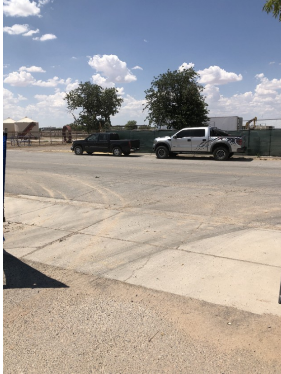
Site Walk Deficiency Photos - West entrance Trackout
