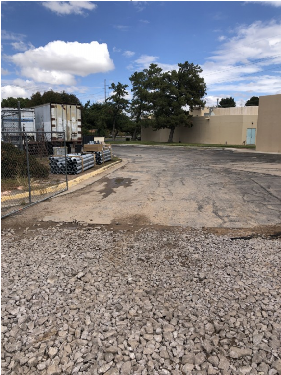
Site Walk Deficiency Photos - NE entrance
