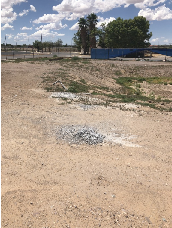
Site Walk Deficiency Photos - Concrete washout on ground SW
