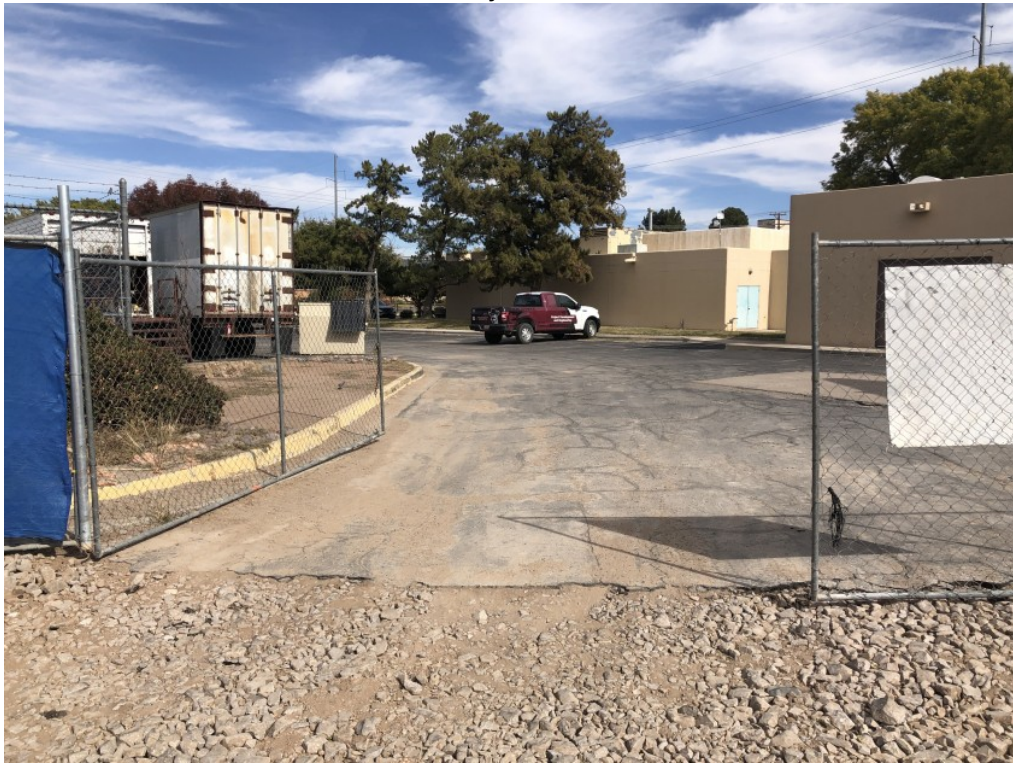
Site Walk Deficiency Photos - NE entrance
