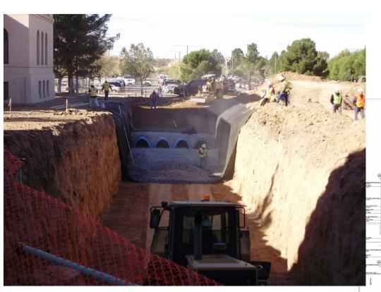
NMSU Center for the Arts; 50K gallons storm water capacity...designed so no runoff leaves the facility!
