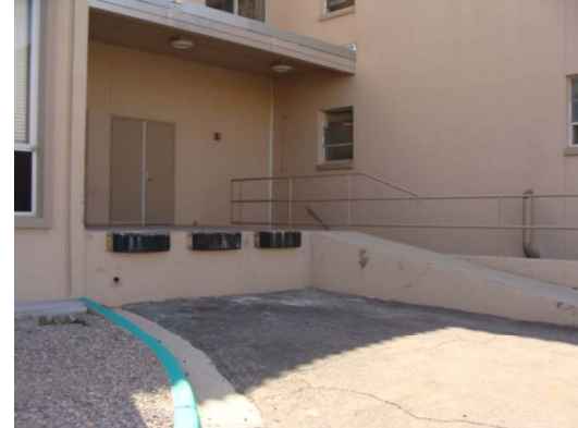
Paint areas for Safety
