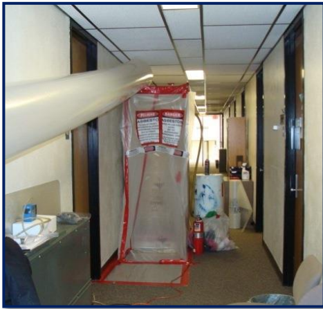
Figure 25: Asbestos Abatement
