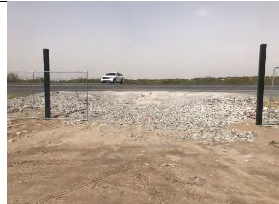
View of rock construction entrance.
