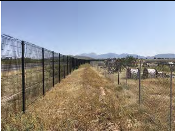
View of earth berm No. 2. Berm is in good shape. entrance.
