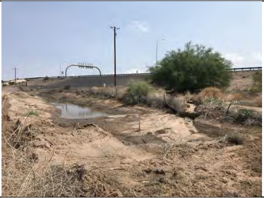
View of drainage swale No. 4. View of entrance point for storm water entering swale.
