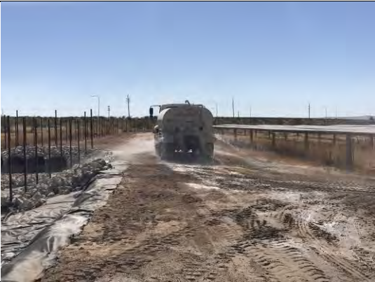
View of water truck spraying perimeter of site with water.
