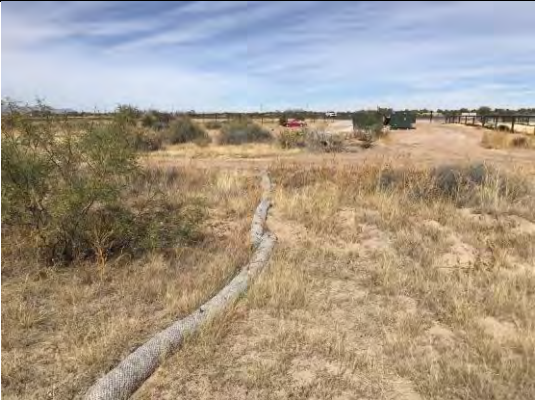
View of straw waddles in place on west side of site.
