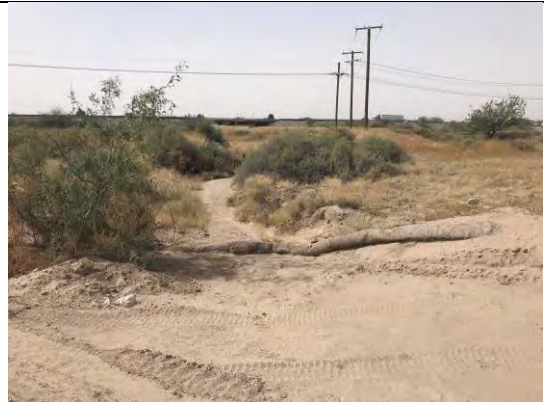
View of straw waddles across discharge point from site.
