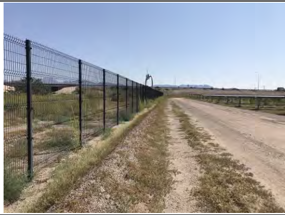
View of earth berm No. 3. Berm is in good shape.
