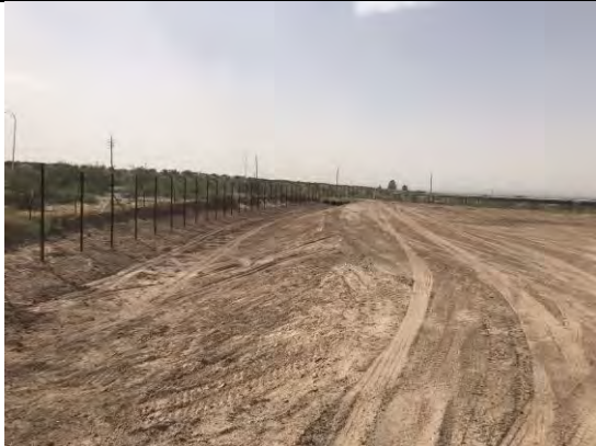
View of drainage swale No. 4. Adjacent earth berm removed, and permanent drainage measure installed.
