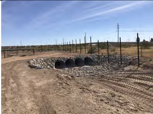
View of drainage pipes entering into drainage swale No. 1.
