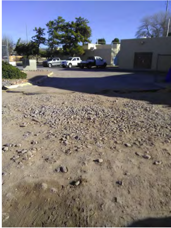
Site Walk Deficiency Photos - NE rock track out pad
