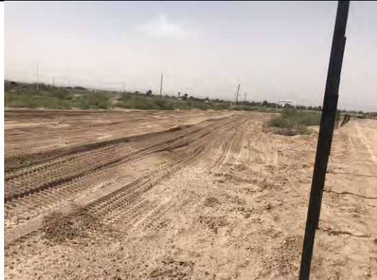
View of drainage swale 3. Swale has been regarded. Earth berm No. 9 removed, and permanent drainage measures installed.
