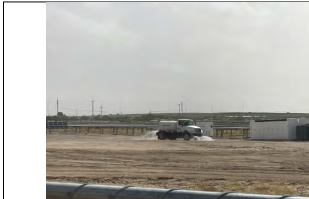
View of water truck placing water on site.
