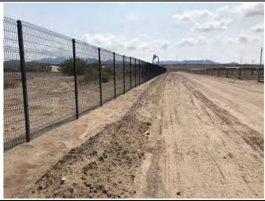
View of earth berm No. 3. No repairs needed.
