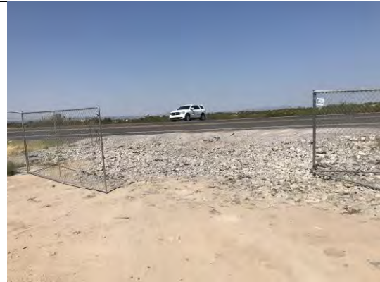
View of rock construction entrance.
