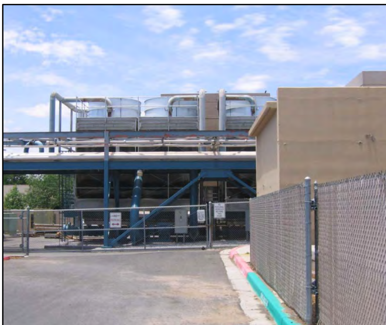
Figure 11. Cooling Towers behind Central Plant (NG-Fired Turbines are within Building on the Right Side).
