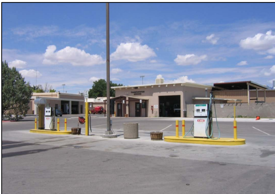
Figure 9. Fleet Maintenance Facility.
