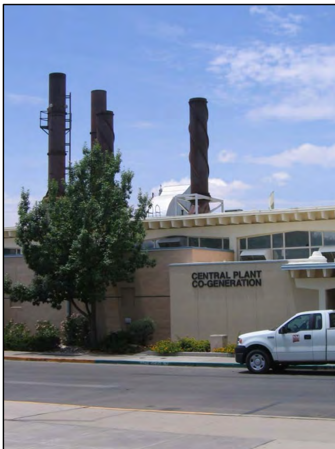
Figure 10. NMSU Central Plant.
