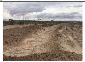
View of drainage swale No. 2 on south side of site. Area is wet where storm water entered swale.
