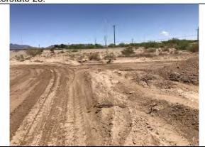
View of earth berm No. 6. Minor repairs needed on east end.
