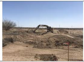
View of Affordable Solar excavating drainage swale No. 4 on east side of site adjacent to Interstate 25.
