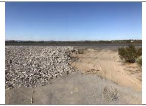
View of temporary stabilized construction entrance. Dirt View o driving area should be removed and berm extended to limit repair. use of non-construction entrance area.
