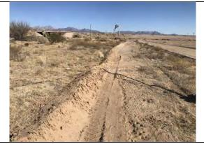
View of exposed cable in Earth Berm No. 2. Cable should be buried or removed.
