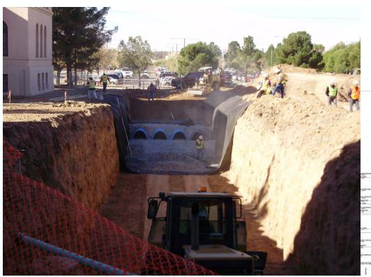
NMSU Center for the Arts; 50K gallons storm water capacity...designed so no runoff leaves the facility!
