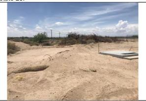
New berm installed connecting south end of earth berm No. 1 to north end of straw waddles.
