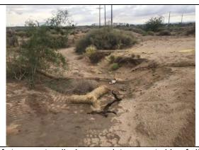
View of storm water discharge point on west side of site. Sediment needs to be removed and waddles repaired.
