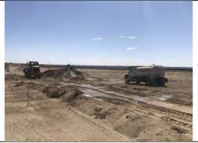
View of water truck spraying stock piled material and area adjacent to excavation of drainage swale No. 4.
