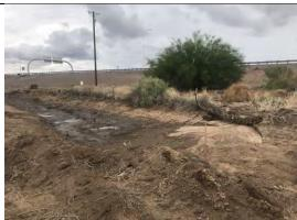
View of drainage swale No. 4 on east side of site. Note where storm water entered berm.
