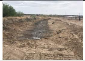
View of drainage swale No. 4 on east side of site adjacent to I-25. All storm water entering site was contained in swale.
