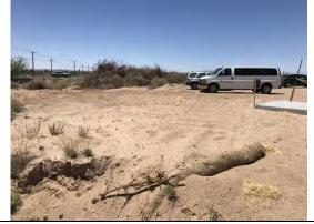
Area where berm is needed to connect south end of EB 1 to north end of straw waddles.
