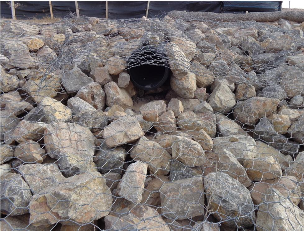
**Located along Arrowhead Drive just west of the Burrell College of Osteopathic Medicine (added during construction of the facility). Outfall discharges from an adjacent detention pond and overflow discharges from Outfall NM035. This outfall discharges into Tortugas Arroyo immediately upstream of the Arrowhead Road concrete culverts.**
