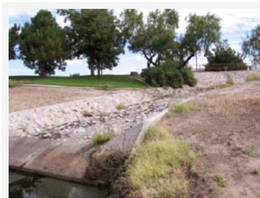
Much of the landscape design on the NMSU campus was created to manage storm runoff. From swales to cuts in curbs, it all serves a purpose - moving storm water away from buildings and to areas where it can absorb into the ground. (Courtesy photo)
